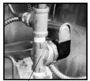
Typical cooling solenoid valve on RK units
