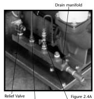
Heat exchanger Pump seal cooling drain line drain line and throttle valve
